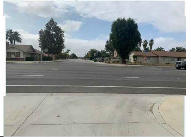
PHOTO 8 View looking south from Emma Lane and Iris Avenue
