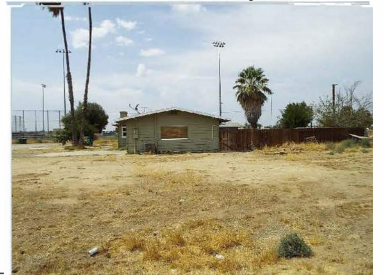
PHOTO 30 Site view at westerly property line looking east
