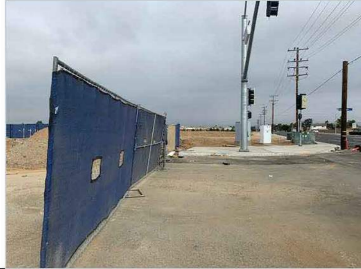
PHOTO 10 View at Santiago Dr. and Perris Blvd. looking north
